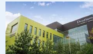
덴티움 Clean Room / GMP
